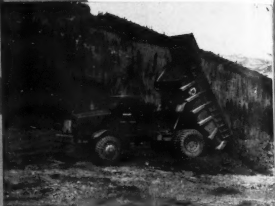
Building a road in the mountains of Colorado—this "Euc" is dumping 15 tons of fill material.
